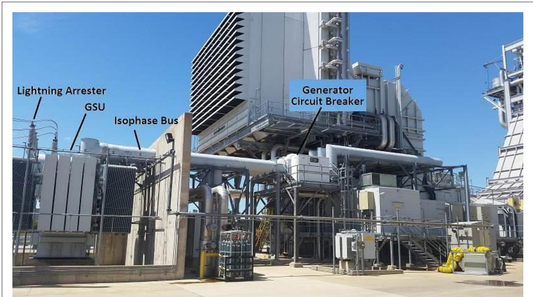
Figure 13: Transmission to IPB, Left to Right.
