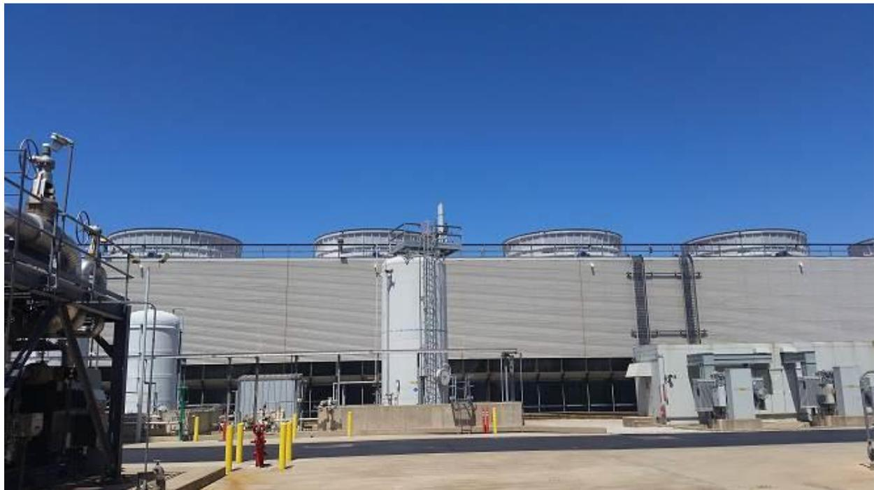
Figure 16: Generating Plant Cooling Towers and Water Treatment Skid.
