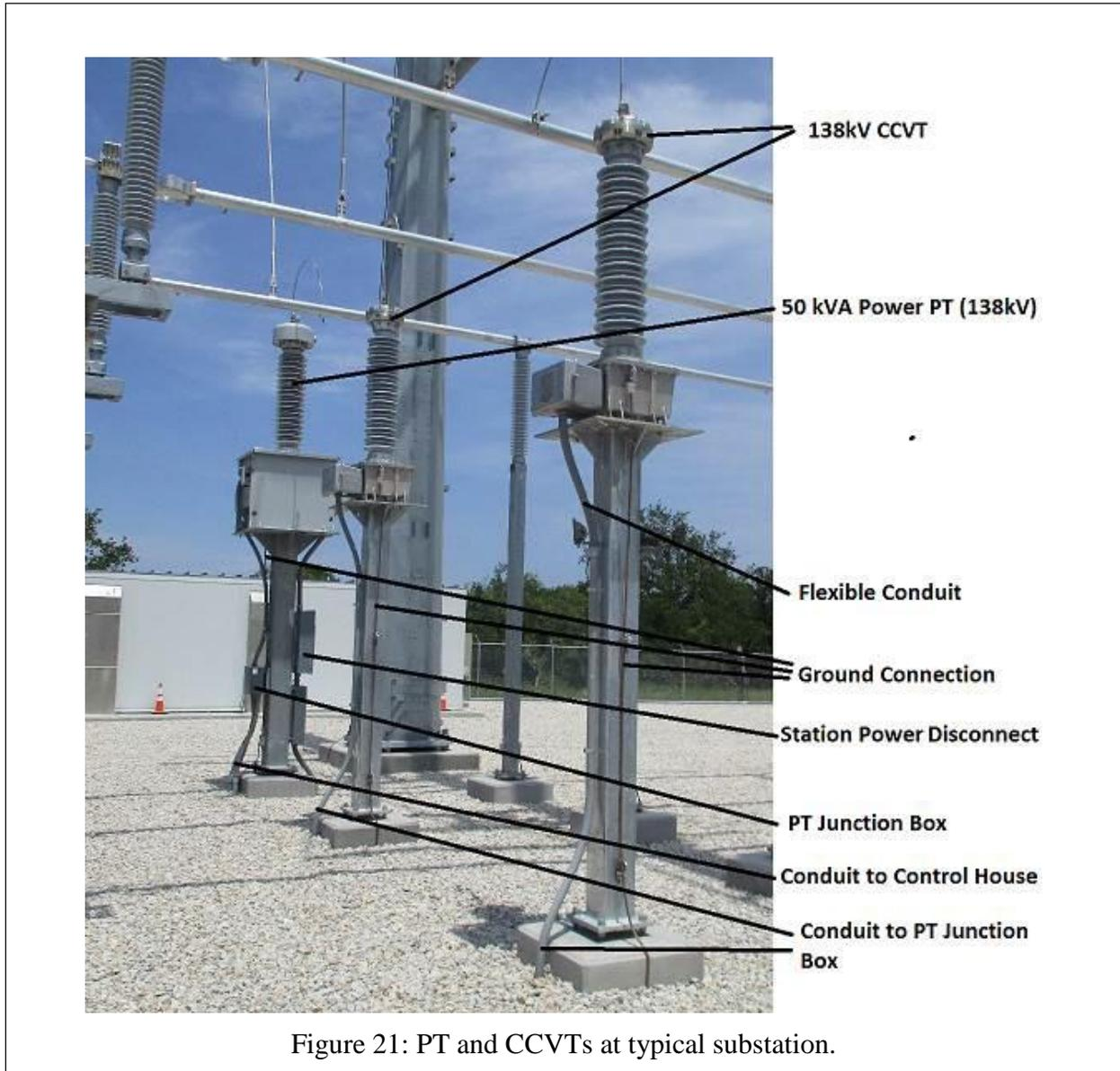
Figure 21: PT and CCVTs at typical substation.
