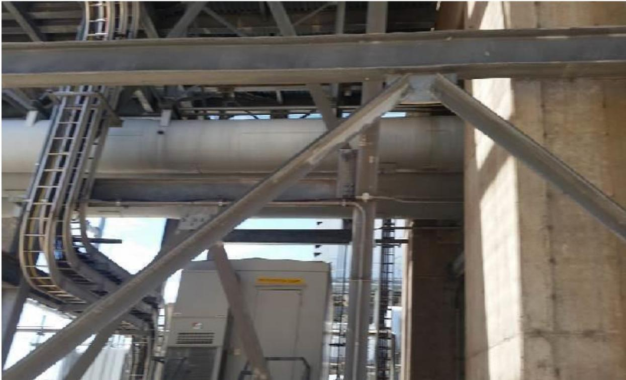
Figure 14: Isophase Bus and Cable Trays.
