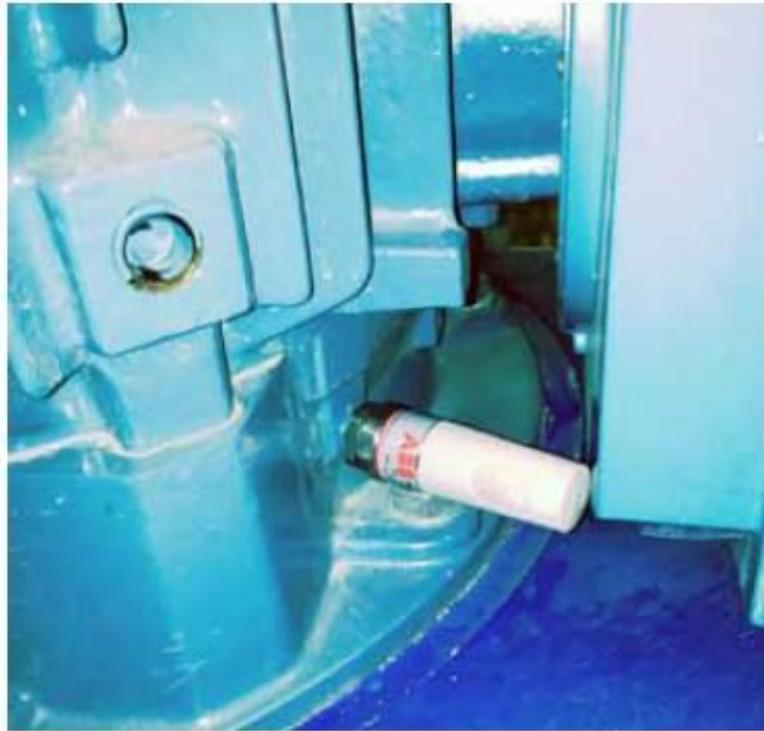
Figure 27: Example of wireless, battery powered generating plant transducer. Approx. 4" long threaded directly into boiler. (ABB WinMon100 Wireless Vibration and Temperature Sensor).
