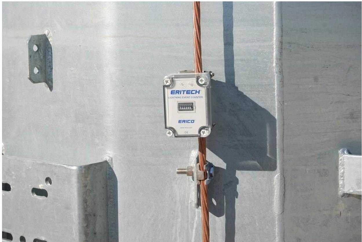
Figure 22: Close up of ground strap with lightning counter.
