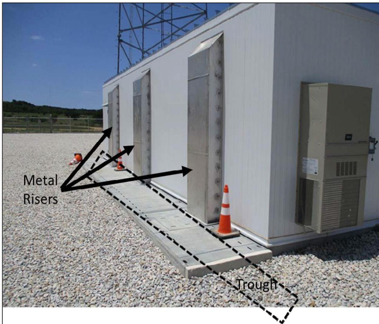
Figure 23. Example of Trough and Metal Risers into Control House.
