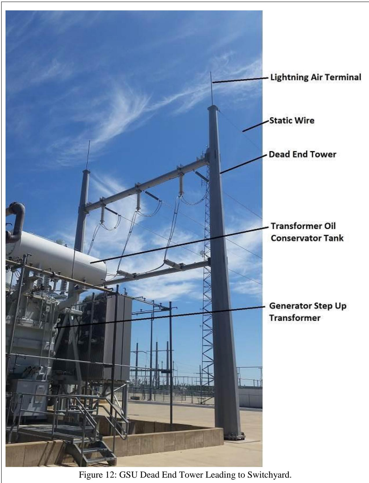
Figure 12: GSU Dead End Tower Leading to Switchyard.
