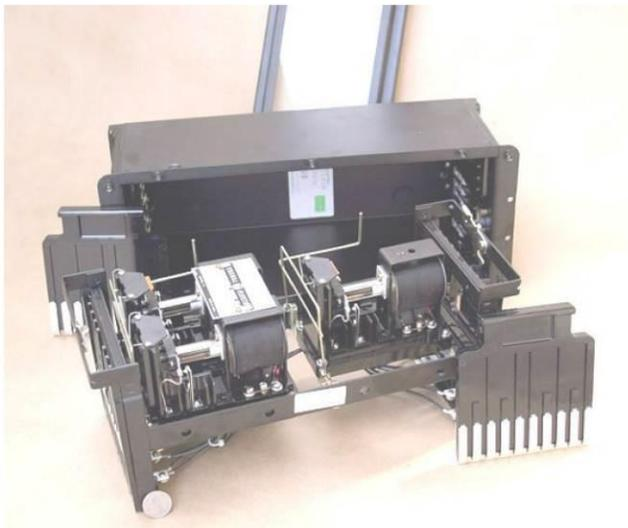
Figure 7-8. GE-PJC electromechanical overcurrent relay.
