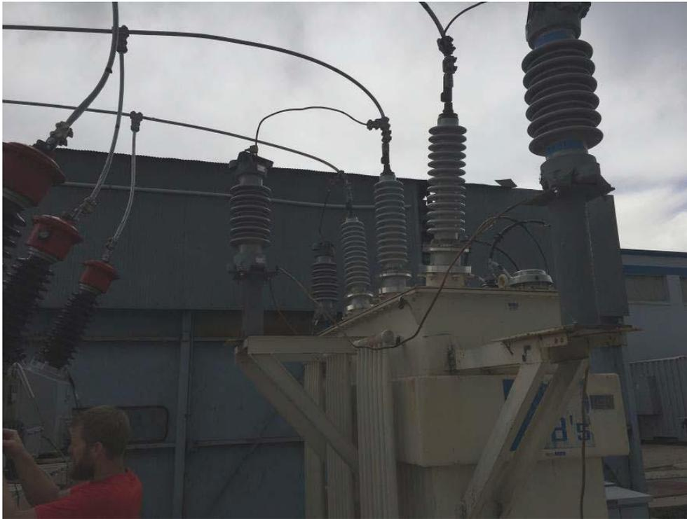
Figure 26. 69 kV Transformer with Lightning Arresters.
